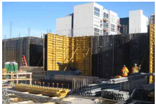
View of the exterior wall formwork, level two of the east block, March 2014.
